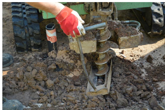
Ground drilling or soil sampling at Valmiera site Photo: Liga Biezina
